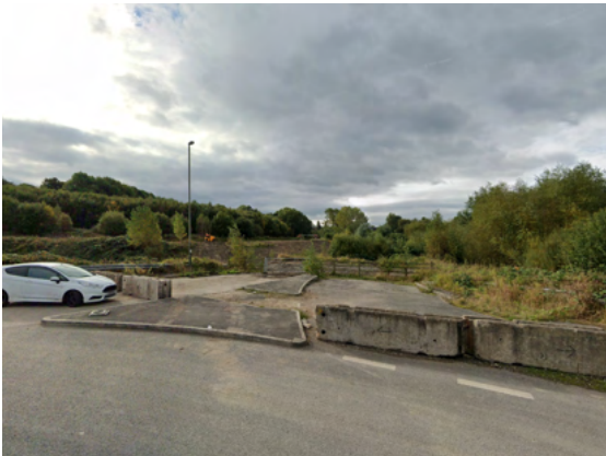
Future CSRR connection point
