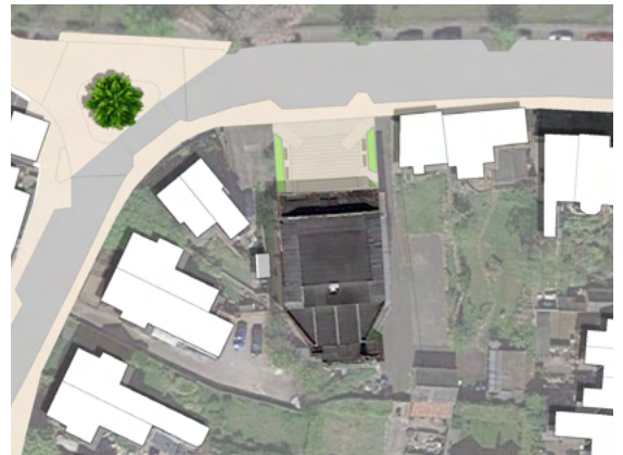
Regal Cinema aerial view
