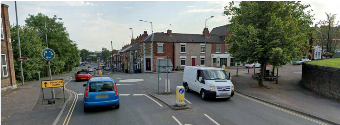
Existing Duke Street Roundabout
